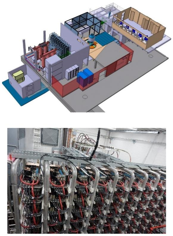
Fig. 1.6.1: CAD view of FULGOR teststand and installation of CW modules.
